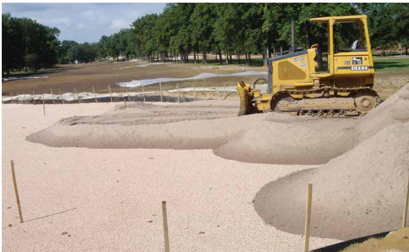
Greens construction typically follows the specifications laid out in the USGA's "Recommendations for a Method of Putting Green Construction" or the University of California Cooperative Extension's "The Sand Putting Green: Construction and Management."
