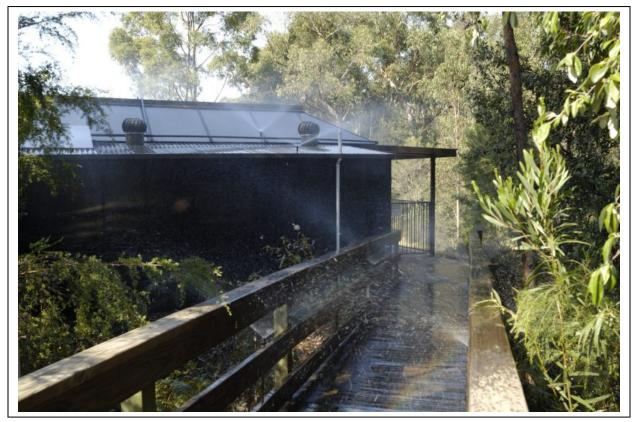
**Figure 6. External sprinklers.** As a wildfire approaches, external sprinklers wet the structure at risk, the surrounding environment, and increase the local humidity to prevent ignition. Photo: A conference center in New South Wales, Australia.
