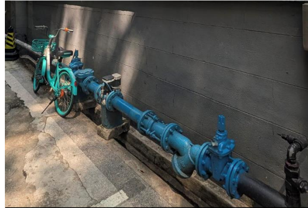
Installed outside old Villa now Starbucks is Model: Hzfengda SCL-61D5 100mm Ultrasonic Water Meter . Flow specs: Q3 = 100 m 3 /h IP68 rating, LCD electronic display with QR code and serial number with External communications module mounted beside the meter
