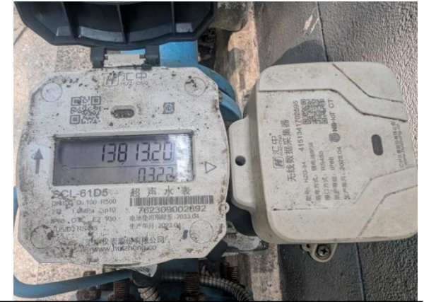
Installed outside old Villa now Starbucks is Model: Hzfengda SCL-61D5 100mm Ultrasonic Water Meter . Flow specs: Q3 = 100 m 3 /h IP68 rating, LCD electronic display with QR code and serial number with External communications module mounted beside the meter
