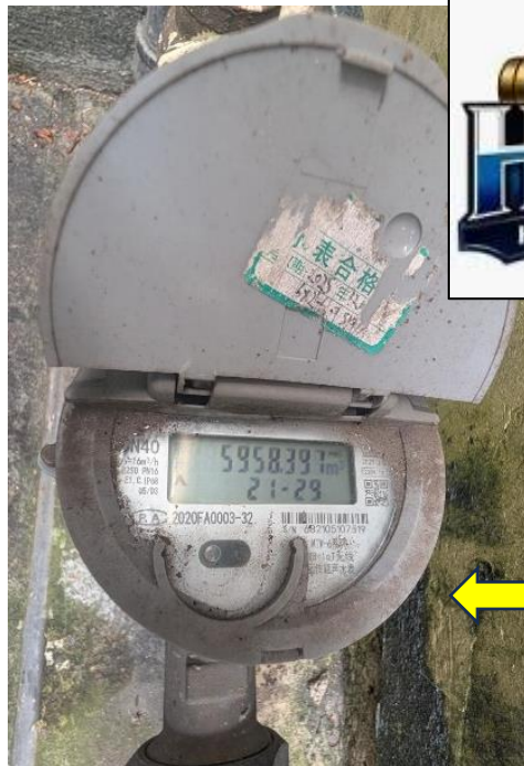
Installed is a unknown Chinese made 40mm Ultrasonic Water Meter with a flow max of 16m 3 /h, battery powered LCD electronic display with a QR code and barcode. Manufacturing approval CPA 2020F.
