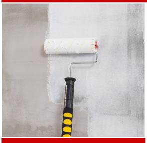
BOND ALL INTERIOR is an interior grade, water based, surface bonding agent applied prior to placing new plaster and Portland cement based mixes over masonry, concrete, brick, block, stone, plaster, drywall, wonderboard, precast concrete, wood, tile and EPS board.
