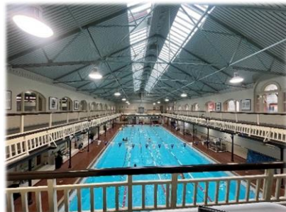
The Melbourne City Baths -1904. We could not locate water meter.
