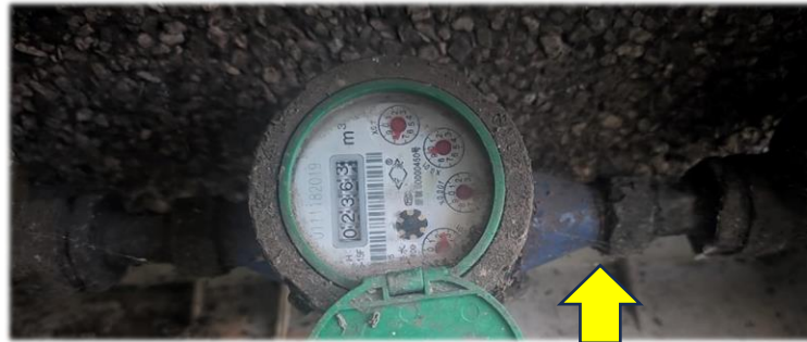
A Xinhai (新海牌) 15 mm domestic Multi-Jet Water Meter is found inside the enclosure.
