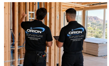
New Construction Low Voltage Pre-Wiring
