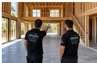
Low Voltage Pre-Wiring Installation
