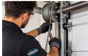
Garage Door Cable Repair
