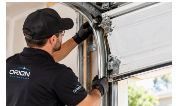
Garage Door Track Repair
