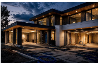
New Construction Low Voltage Installation
