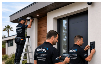
Security Camera and Intercom Installation
