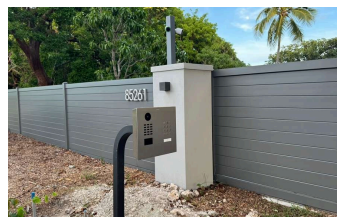
Residential Gate Intercom Installation
