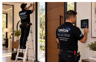
Alarm and Intrusion System Installation
